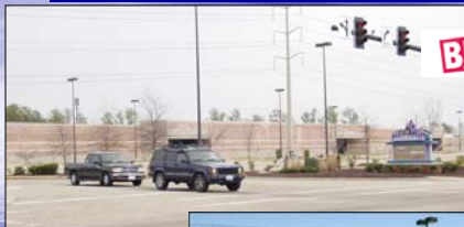
Power Plant - Hampton
