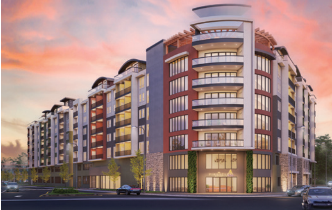
The Pinnacle on 31st Street - Virginia Beach, VA
